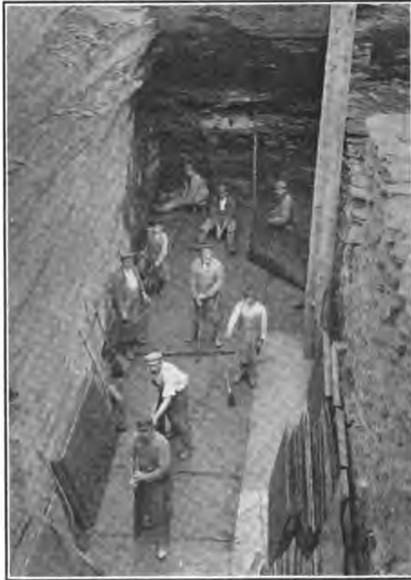
FIG. 1626. — Quarry in the Posidonia slates of the upper Lias, at Holzmaden in Württemberg, Bavaria. The quarry is only 7 meters in depth, the slabs quarried are 20 cm. in thickness and represent the bedding of the series. The left wall of the quarry is a natural joint, the right side is made of discarded fragments. At the point marked + on the rear wall the specimen represented in the succeeding figures was found. In 1911, more than 25 such quarries were in operation in this region. These furnish during the year about 100 specimens of saurians of which on the average only 10 are sufficiently perfect to warrant preparation. (Photo by courtesy of Bernard Hauff Holzmaden-Teck.)
